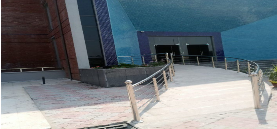
Ramps Provided for handicapped Peoples to easily access to Building
